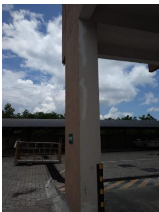
Figure 4. Patch repair of cracks in columns
