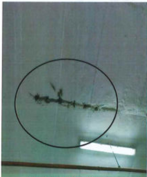
Grouting on RC slab
