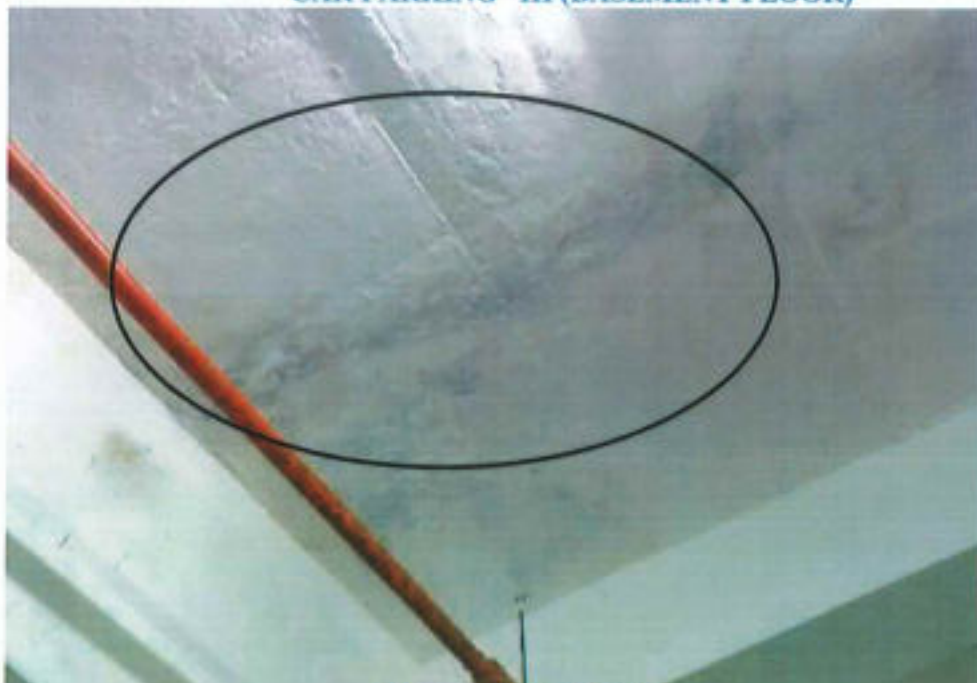
Dampness on RC Slab
