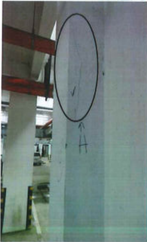
Crack on staircase wall
