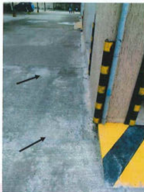
6mm metal plate (L-shape) provided at expansion joint region between parking area and tower-B & C
