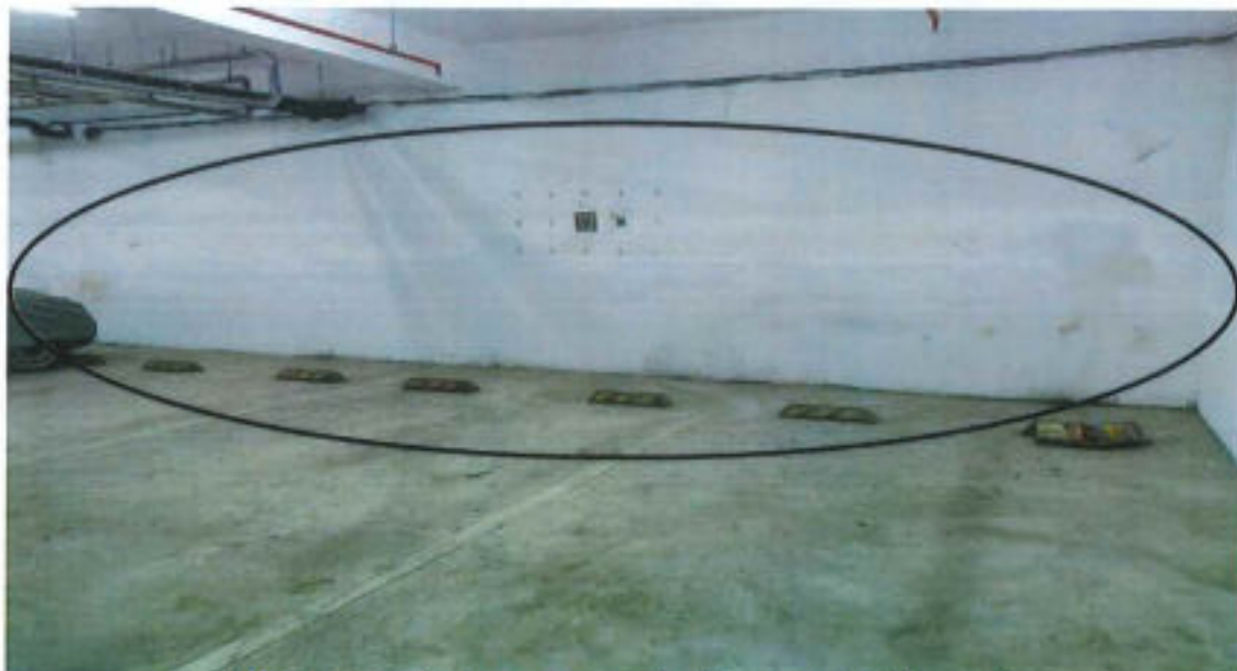
Dampness, minor seepage and patchup on retaining wall
