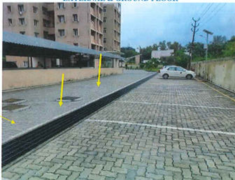
Rain water trench at south face away from retaining wall
