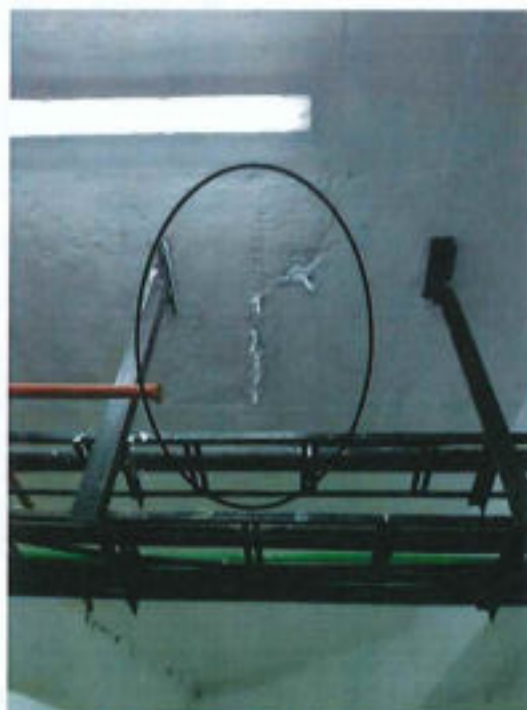
Grouting on RC slab
