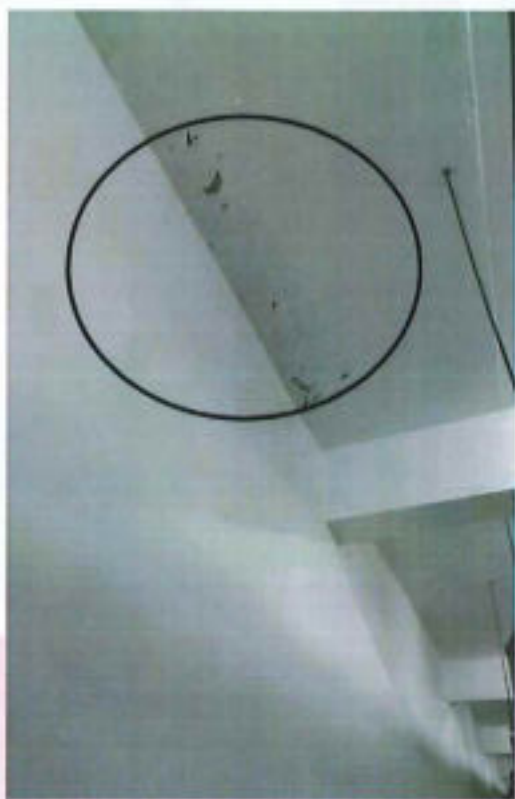
Peeling of paint on RC Slab
