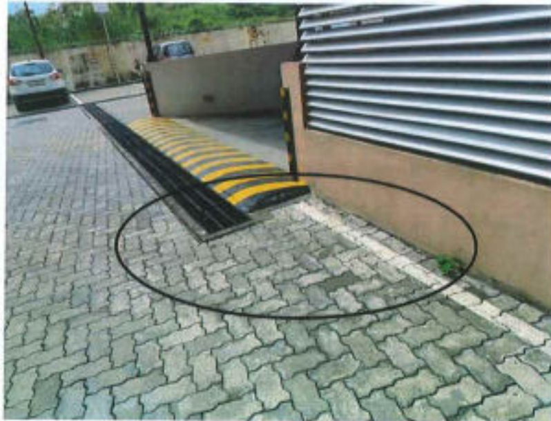
Gap between ramp wall and paver block
