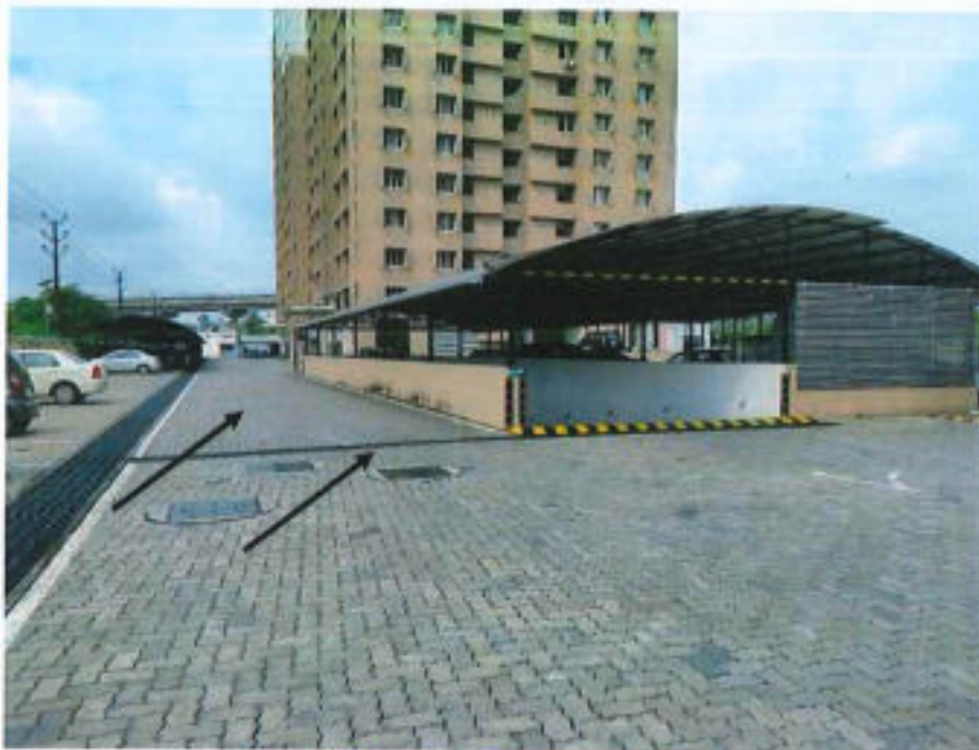
Gap between ramp wall and paver block
