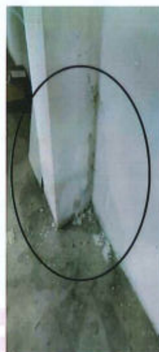
Crack on RC column
