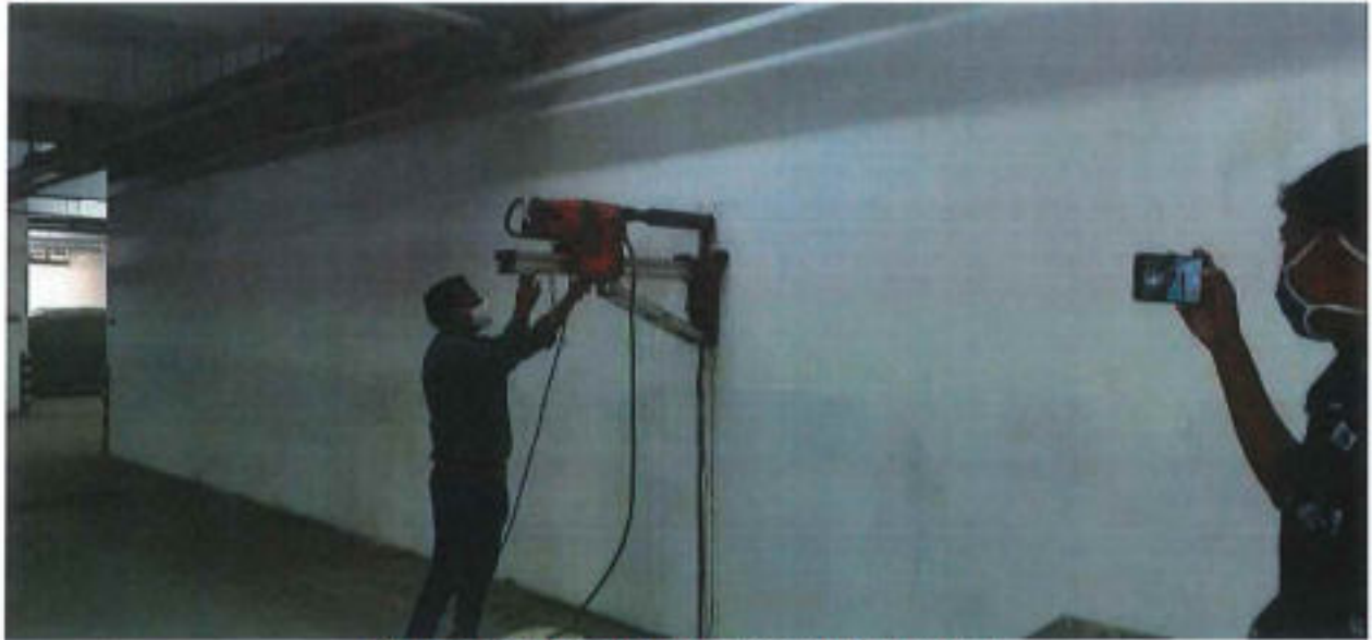
Extraction of concrete core sample in progress
