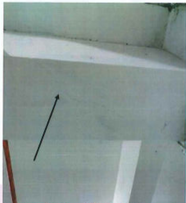
Crack on RC beam bottom
