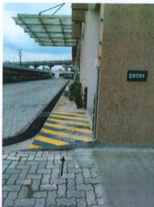
6mm metal plate (L-shape) provided at expansion joint region between parking area and tower-B & C
