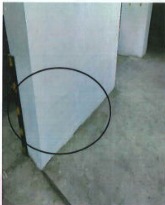
Patchup work on RC column
