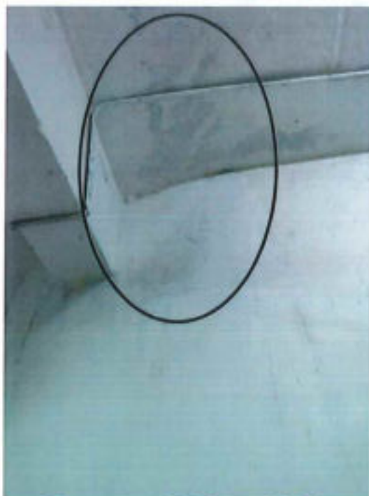
Dampness on RC Beam & Slab
