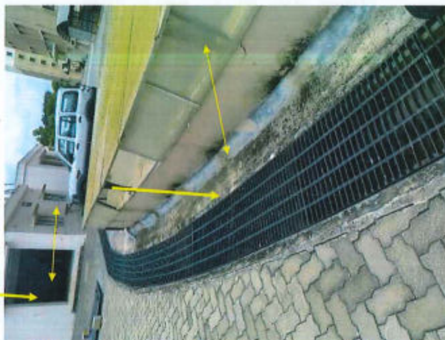
Rain water trench at northwest face nearer to retaining wall
