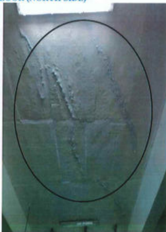
Grouting work on RC slab
