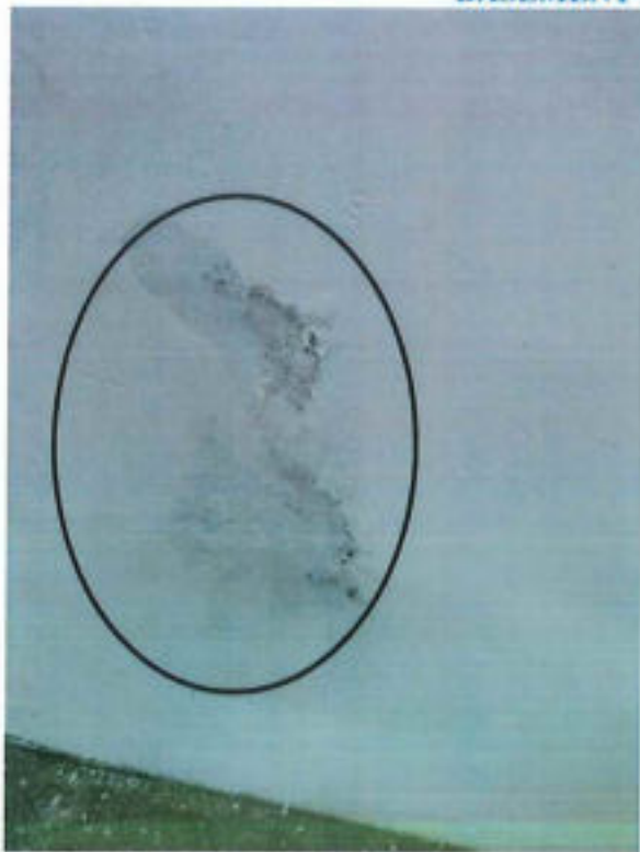
Dampness on Retaining wall
