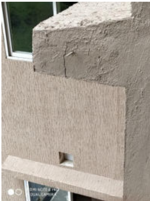
Figure 12. Cracks in shade
