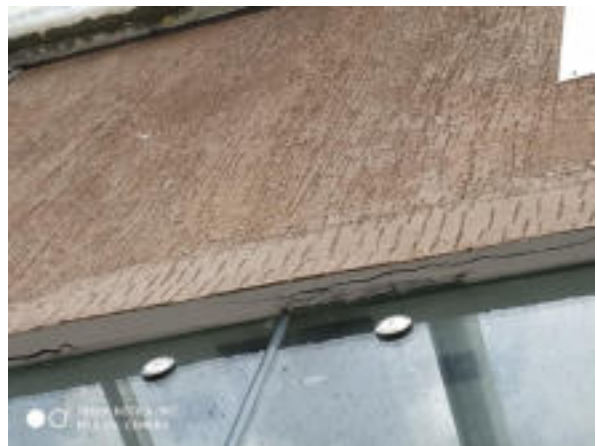
Figure 6. Reoccurrence of cracks in the already repaired beams
