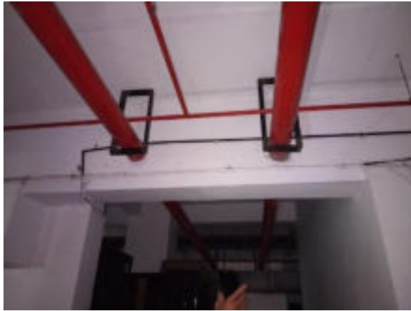
Figure 2. Improper cutting of the beams for fire pipes
