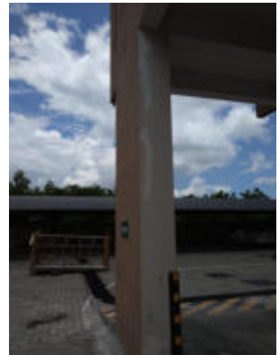
Figure 5. Improper repair of cracks in columns with filler material
