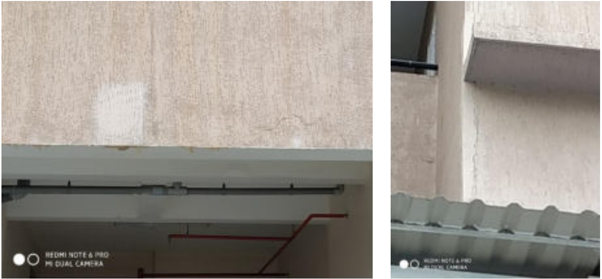
Figure 9. Occurance of cracks in the visinity of already repaired portion
