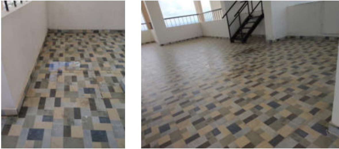
Figure 13. Water is getting stagnated in the floor
