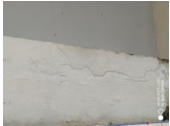
Figure 4. Cracks on the beams due to corrosion
