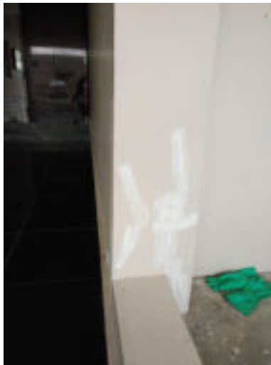
Figure 5. Improper repair of cracks in columns with filler material
