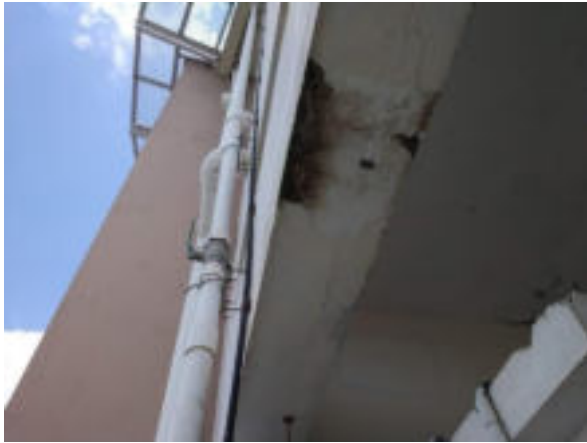
Figure 4. Cracks on the beams due to corrosion
