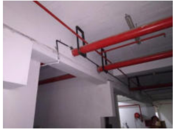
Figure 2. Improper cutting of the beams for fire pipes
