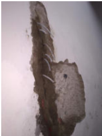
Figure 1. Repairing of the leaking portions in the basement
