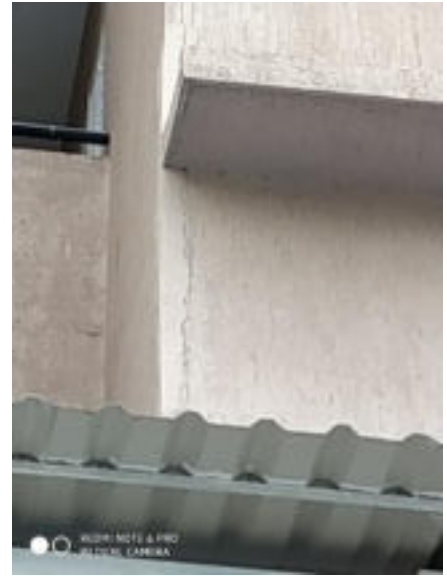
Figure 9. Occurance of cracks in the visinity of already repaired portion
