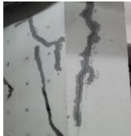
(d) Cracks reappeared in patch-repaired shear wall
