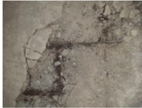
(b) Disintegrated concrete and severely corroded rebars
