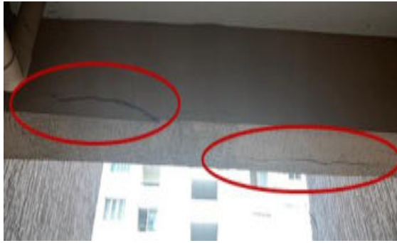
(a) Multiple longitudinal cracks in the side face and soffit of a beam
