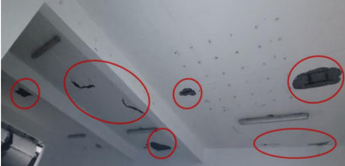
(a) Cracked, spalled and exposed corroded rebars at various locations
