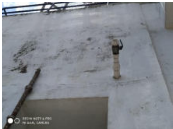
Figure 3. Dampness in the walls and water tank walls
