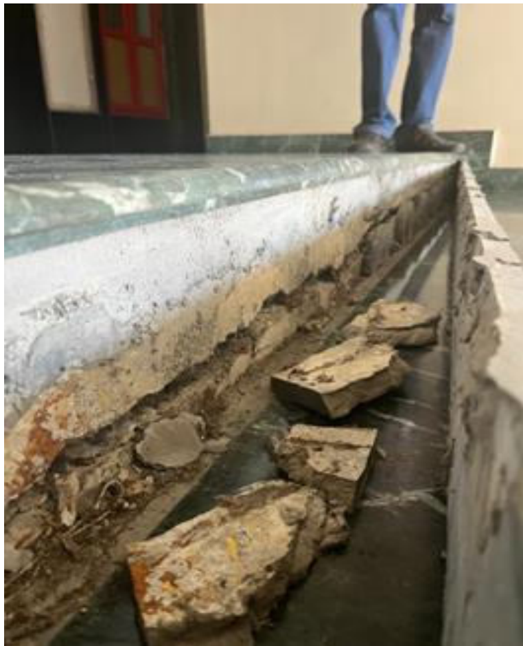
(b) Disintegrated concrete and corrosion stains
