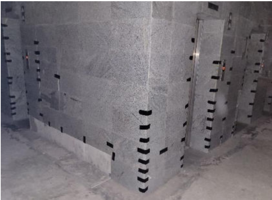
(b) De-bonded cladding inadequately held using tape around the entire elevator area in the basement
