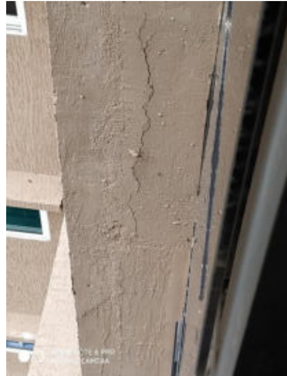
Figure 11. Cracks in columns due to corrosion of reinforcement
