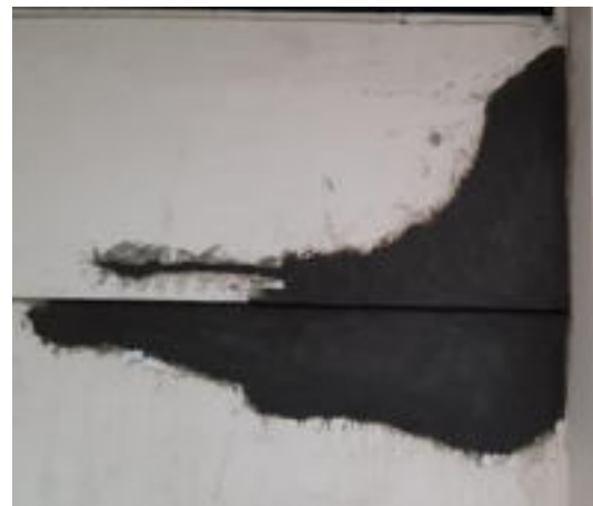
(f) Cosmetic repair of spalled region
