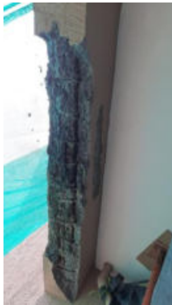
(b) Spalled and exposed corroded rebars
