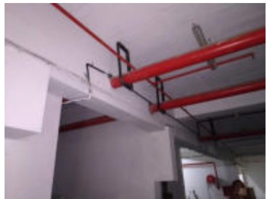
Figure 3. Fire pipes passing through the beams (the consequences must be checked by a structural consultant)
