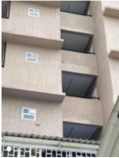
Figure 7. Repaired beams on the balcony of almost every floor and many shades
