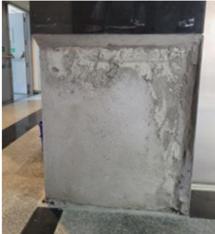
(a) Cosmetic repair of spalled region of the shear wall near elevator
