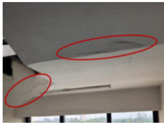
(g) Cracks at various locations
