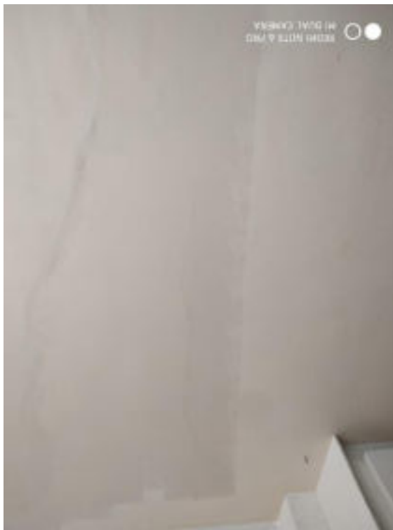
Figure 10. Reoccurance of cracks in the repaired portions
