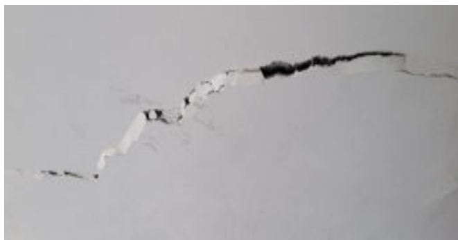
(c) Cracked and delaminated concrete
