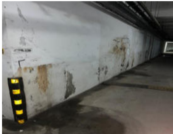
(d) Flaked paint and corrosion stains on retaining walls and water leakage
