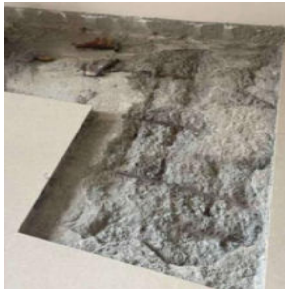
(e) Disintegrated concrete and severely corroded rebars
