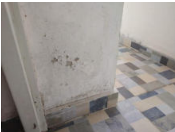
Figure 3. Dampness in the walls and water tank walls
