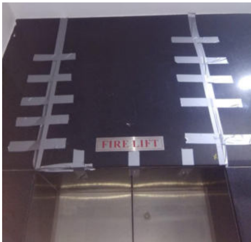
(d) De-bonded granite cladding inadequately held using tape
