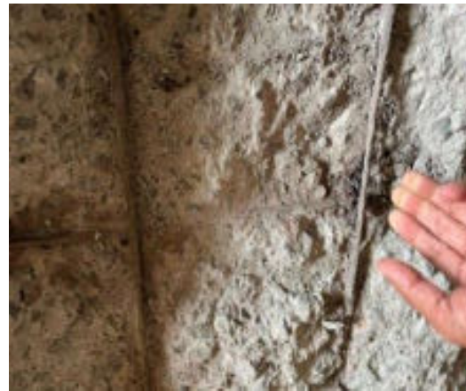
(d) Disintegrated concrete and corroded rebars with significant cross-section loss
