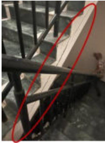
(a) Wide crack in waist slab
