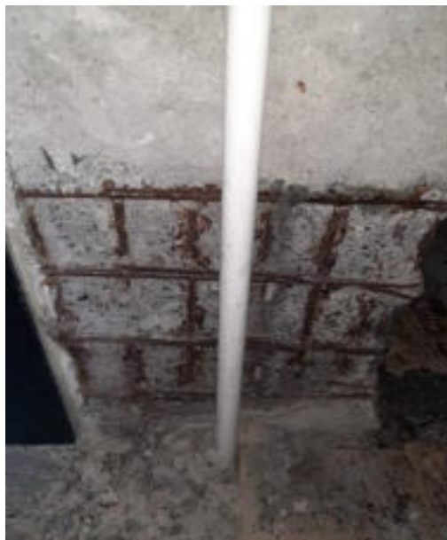
(e) Spalled and severely corroded rebars
