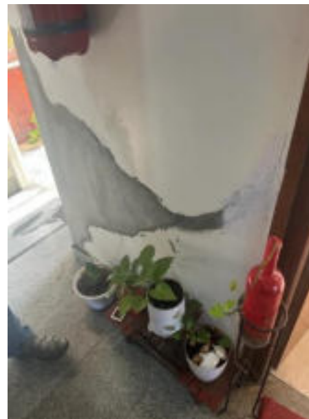
(f) Cosmetic repair of spalled region
