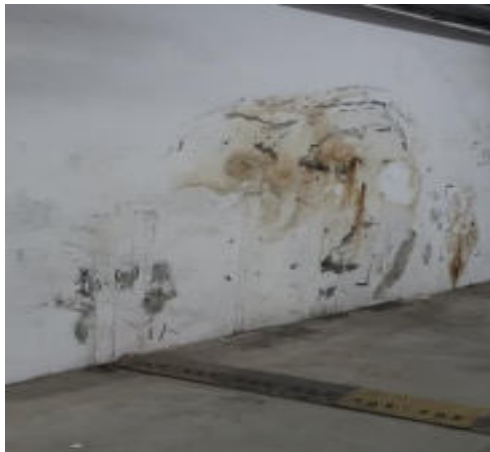
(c) Flaked paint and corrosion stains on retaining walls
