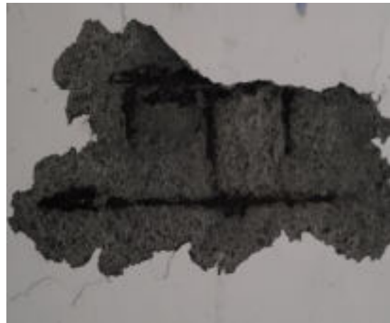
(e) Spalled concrete and exposed corroded rebars
