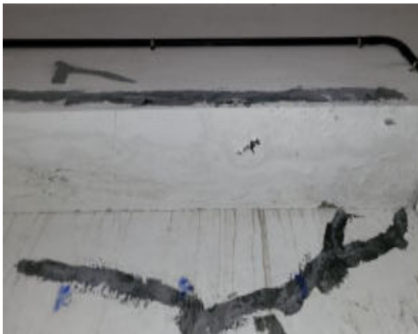
(b) Cosmetic repair of cracks
