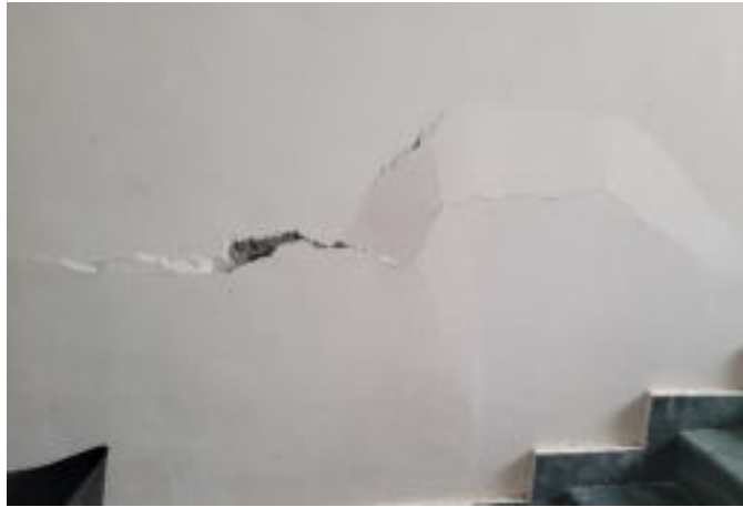
(a) Cracked, delaminated and spalled concrete
