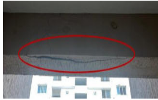
(b) Wide longitudinal crack in the soffit of a beam
