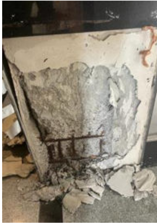
(b) Disintegrated concrete and severely corroded rebars visible after removal of de-bonded cladding
