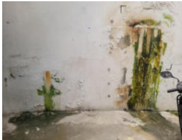
(b) Flaked paint, corrosion stains and algae growth on retaining walls and water leakage
