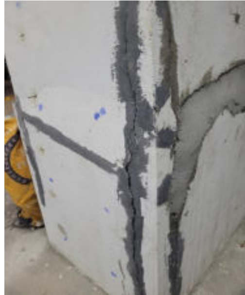
(b) Cracks reappeared in patch-repaired shear wall
