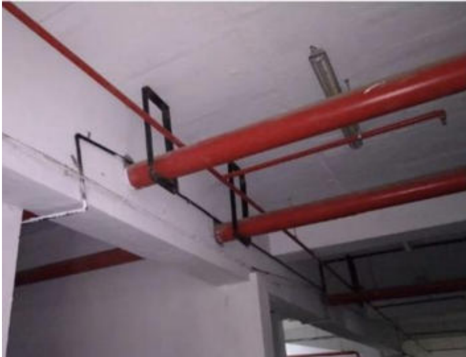
Figure 7 Fire-fighting system pipes passing through the beams
