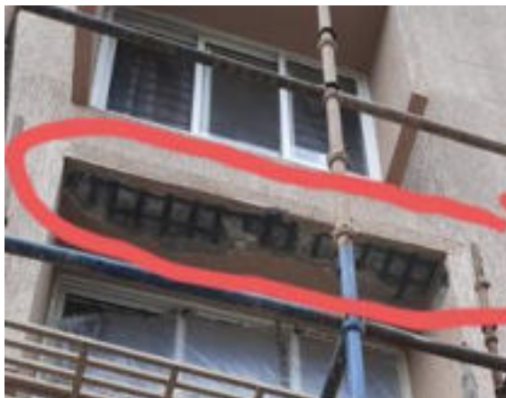
(e) Spalled and severely corroded rebars
