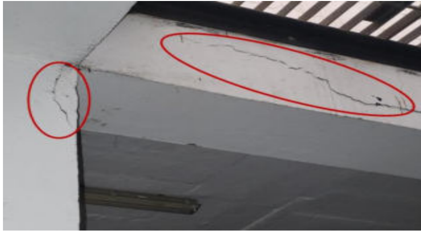
(a) Cracks in the beam-column joint and side face of a beam
