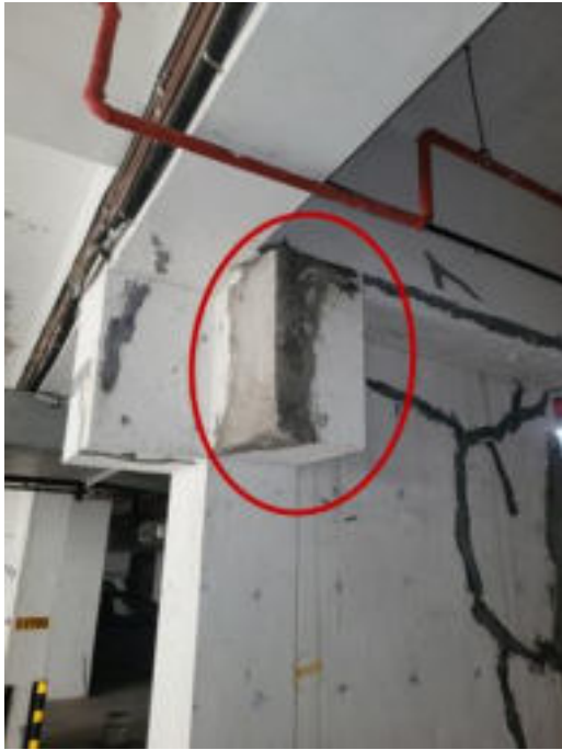
(g) Cosmetic repair of spalled region and cracks
