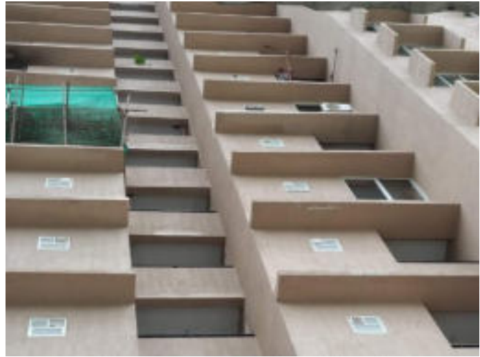
Figure 7. Repaired beams on the balcony of almost every floor and many shades
