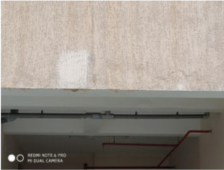
Figure 9. Occurance of cracks in the visinity of already repaired portion
