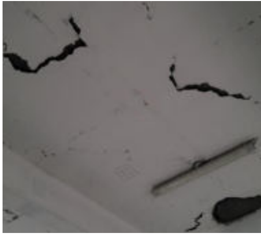
(b) Cracked and delaminated concrete
