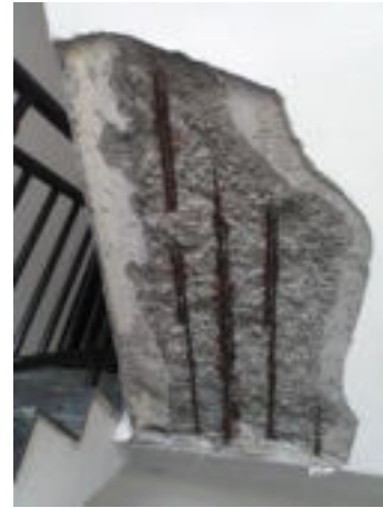
(c) Spalled concrete and exposed corroded rebars
