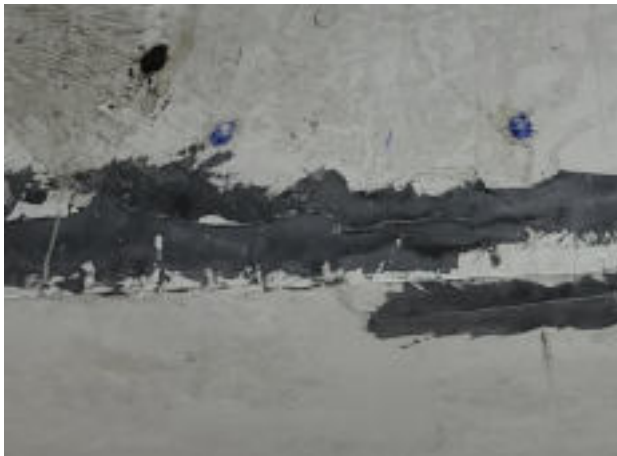
(c) Cracks reappeared in patch-repaired beam
