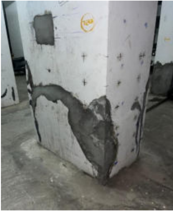
(a) Cosmetic repair of spalled region
