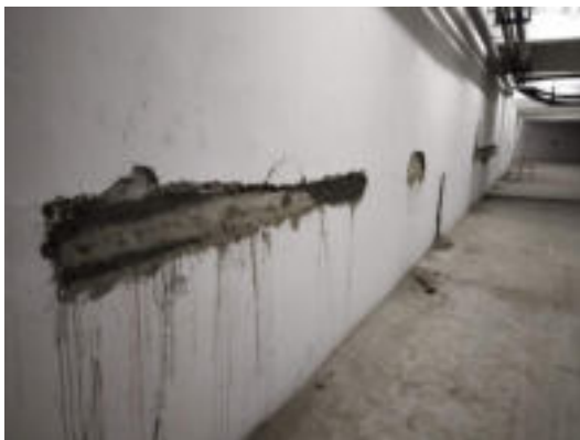
Figure 2. Leaking of basement wall (performance of recent repair must be checked during the upcoming monsoon)
