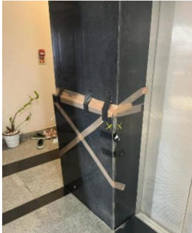
(a) De-bonded cladding inadequately held using tape
