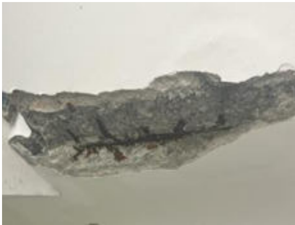
(c) Spalled concrete and exposed corroded rebars
