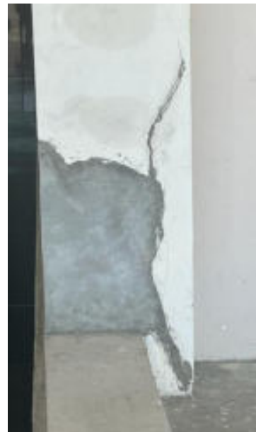
(c) Cosmetic repair of spalled region
