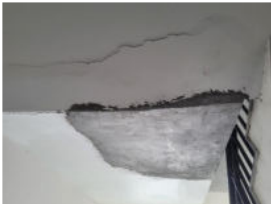
(d) Cracks and cosmetic repair of spalled region
