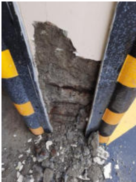
(a) Spalled and corroded rebars
