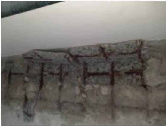
(a) Severely corroded rebars
