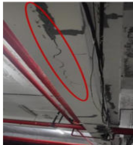
(c) Cracks reappeared in patch-repaired region in beam
