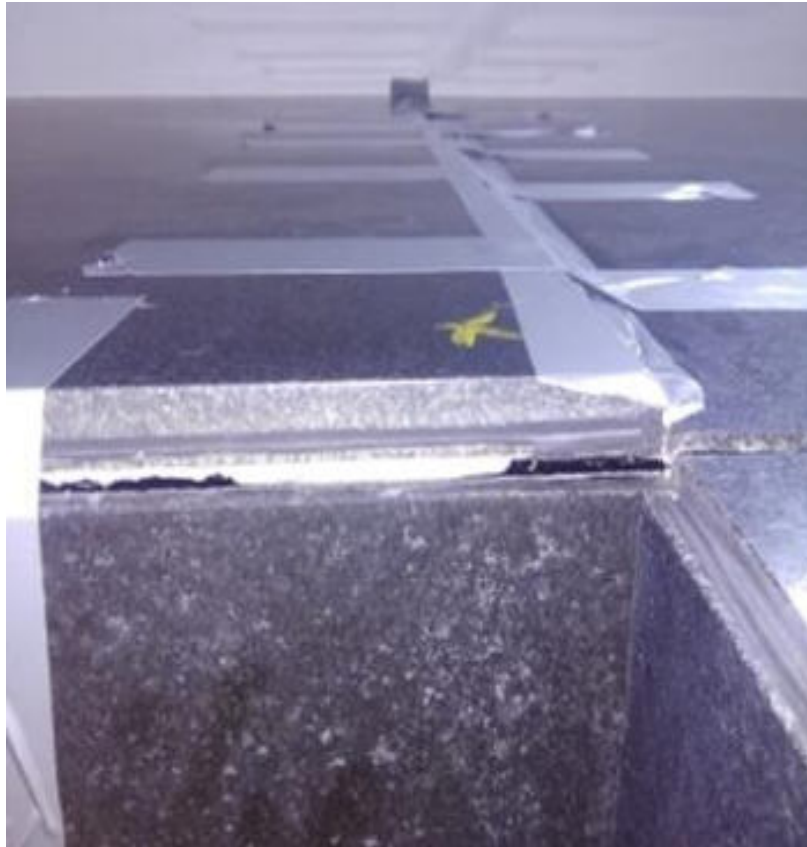
(c) De-bonded granite cladding hanging dangerously above lift door (looking upward)
