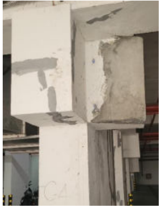
(h) Cosmetic repair of spalled region and cracks
