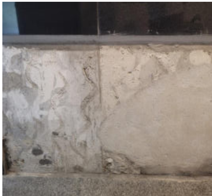
(b) Cosmetic repair of spalled region
