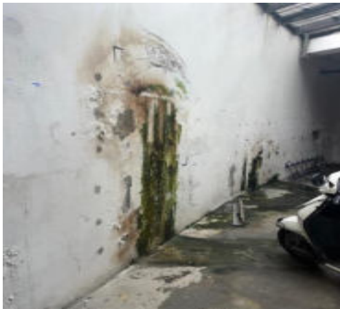
(a) Flaked paint, corrosion stains and algae growth on retaining walls and water leakage
