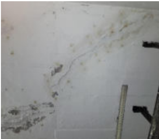
(d) Flaked paint, dampness, corrosion stains and cracks
