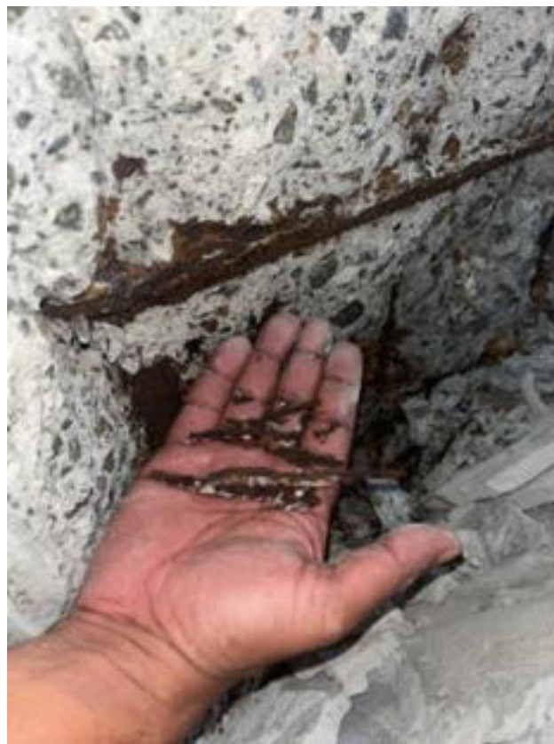
(c) Severely corroded rebars with significant cross-section loss
