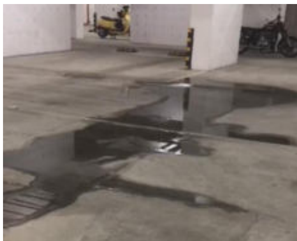
(f) Water leakage during rain
