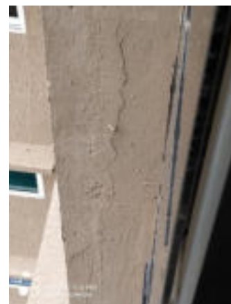
Figure 5. Cracks on patch repaired columns (indicate inadequate repair practice)
