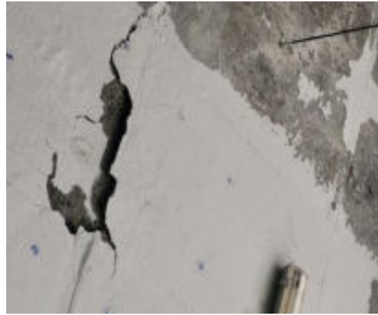
(c) Peeled-off paint, cracked and delaminated concrete
