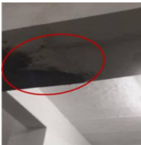
(e) Water dripping from beam and dampness on beam during rain
