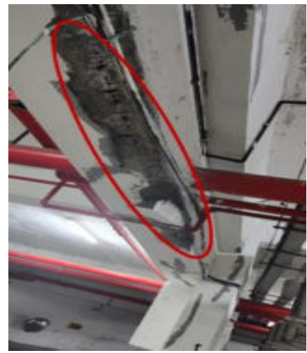
(e) Spalled concrete in beam and patch repairs
