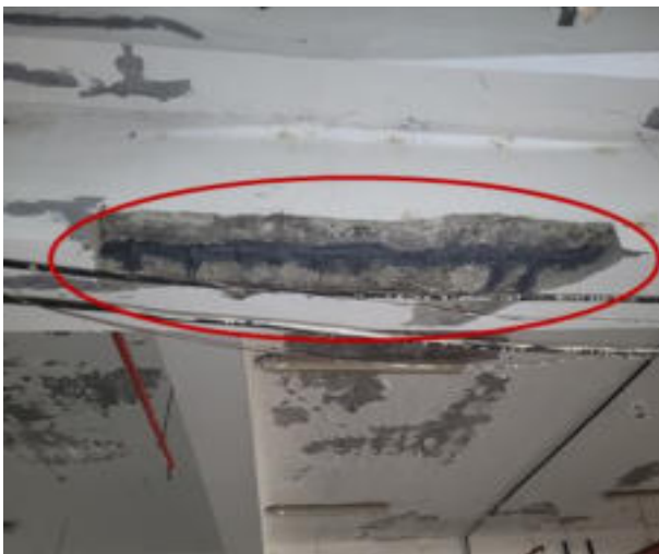
(d) Spalled concrete and cement paste applied over rebar to cover up corrosion of rebar
