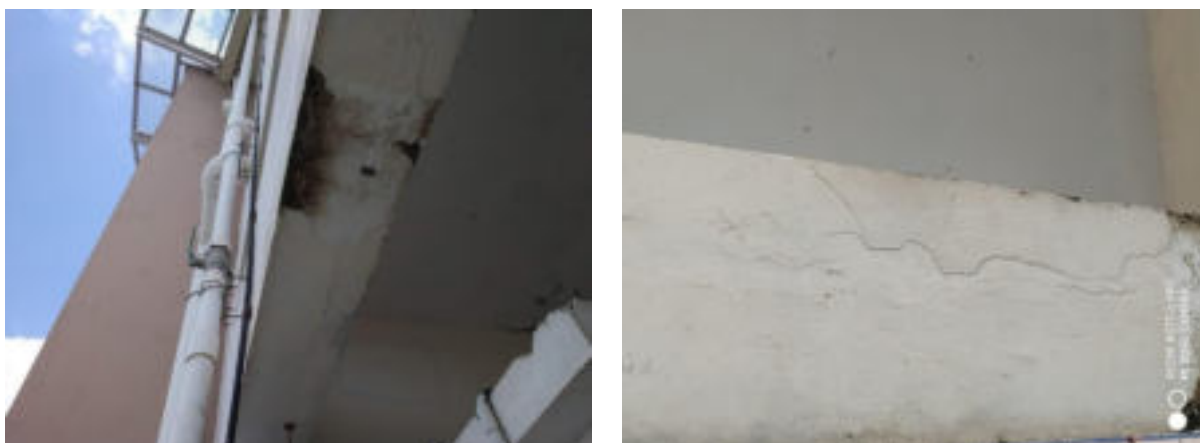
Figure 4. Cracks on the beams due to corrosion
