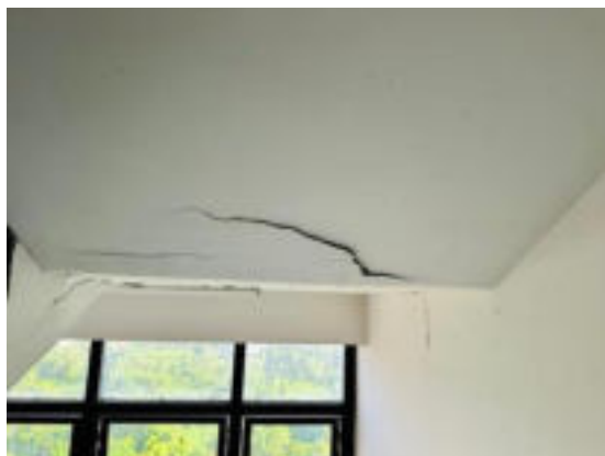
(f) Extensive cracking and delamination
