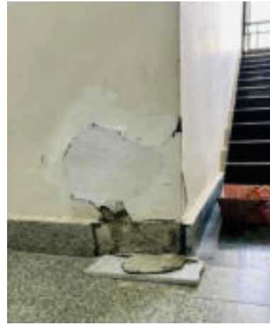
(b) Cracked, spalled concrete with cosmetic repair
