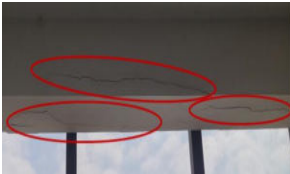
(c) Multiple longitudinal cracks in the side face and soffit of a beam
