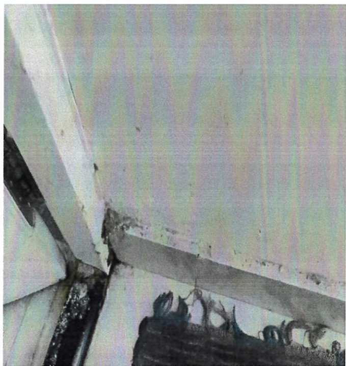
View of dampness/ damp patches/ peeling of paint inside the Flats
