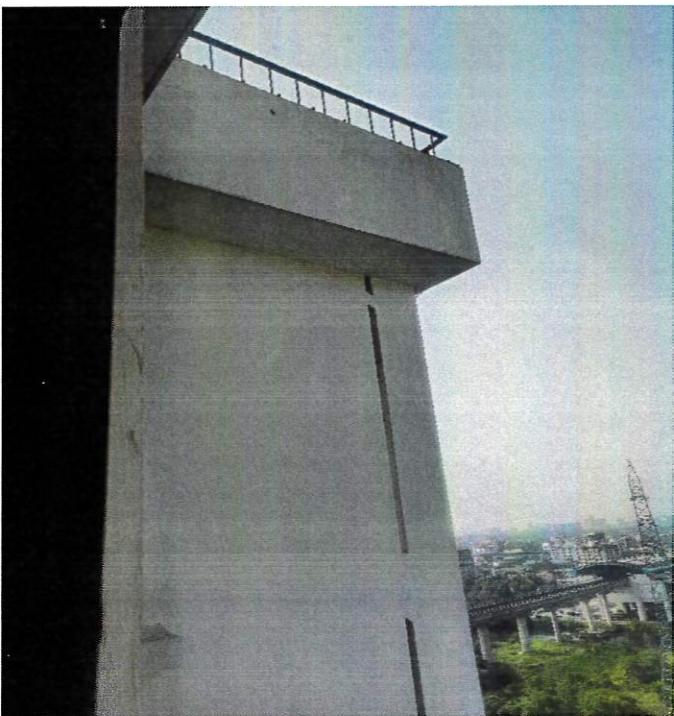
View of cracks in masonry wall
