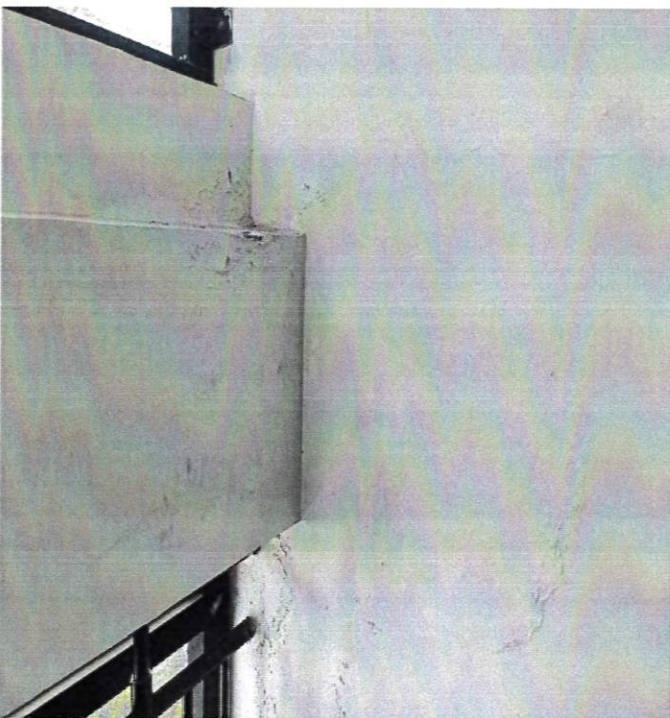
View of dampness/ damp patches/ peeling of paint
