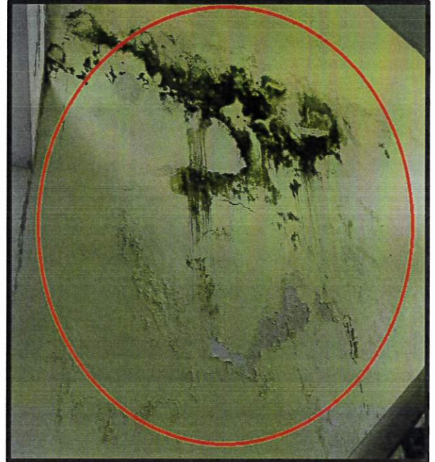
View of Peeling of paint and damp patches in masonry wall at stair case regions
